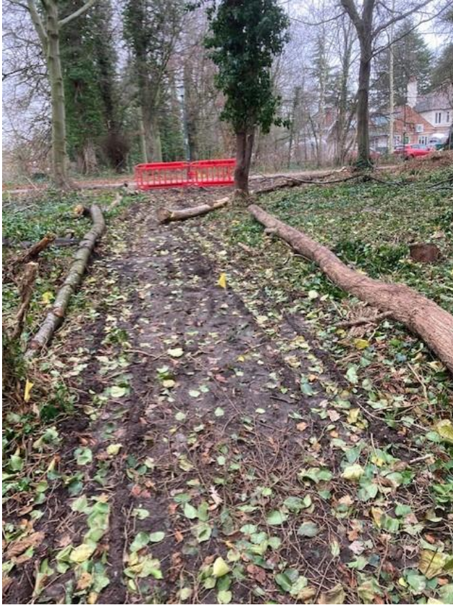
Image of construction of woodland footpaths
