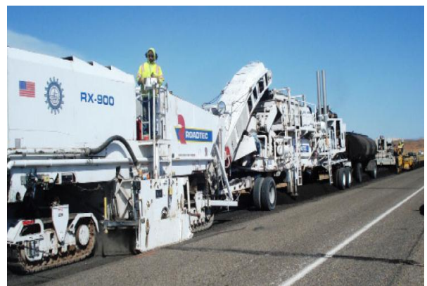
Cold Asphalt Emulsion Mixtures used in recycling an asphalt pavement layer
