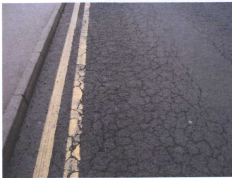
Fatigue Cracking
