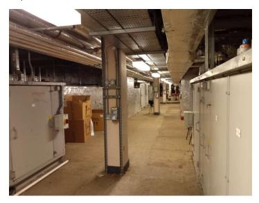
There are also heat recovery run round coils on the 2 lab supply and extract systems which are currently not operating, requiring service/ maintenance, which should reclaim about 50% of the required heat energy. Annual energy saving potential is a very significant 500,417 kWh.
