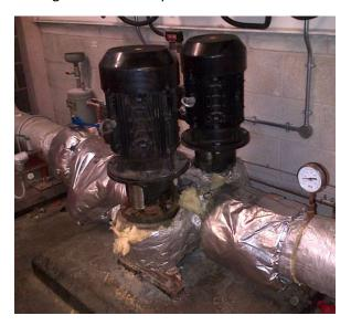
As there are no reheat requirements for humidity control or domestic hot water requirement from this system it is recommended the pumps and boiler are turned off when outside temperature exceed 18°C. This will save significant electrical energy of up to 11,500 kWh and also standing heat losses on the distribution pipework of around 1050kWh.
