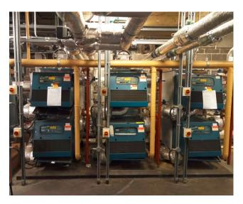
The boilers are due for replacement under the capital backlog replacement programme and should save around 90,000kWh. There was an option to provide additional supplementary heat pumps to provide heating through the mild months of the heating season, however this was ruled out due to the high life time cost per tonne of carbon saved.
