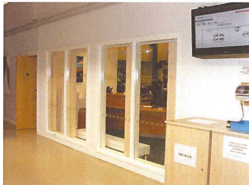
Glazed screen giving borrowed light to office
