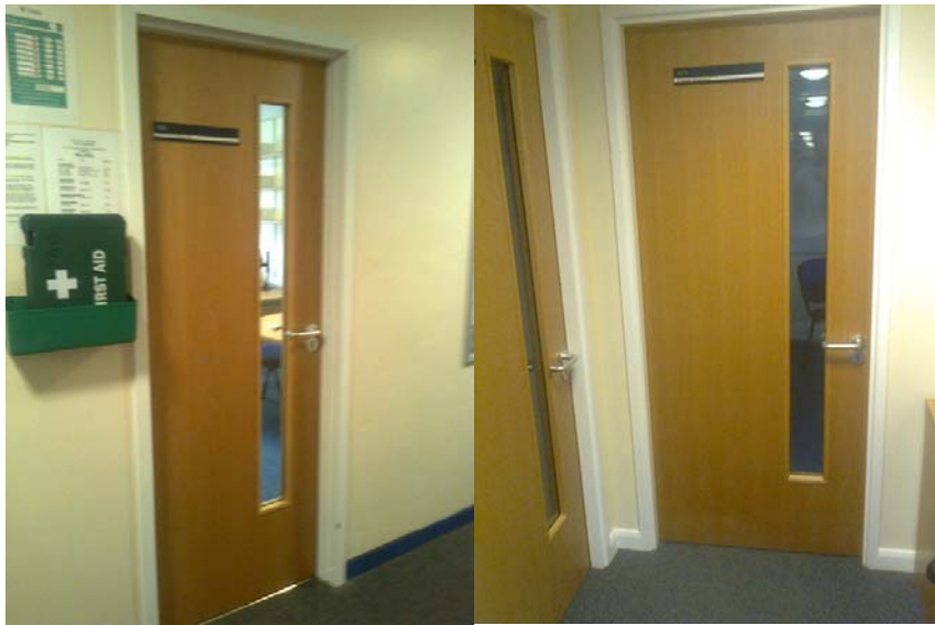
Coates building - New style door leafs.
