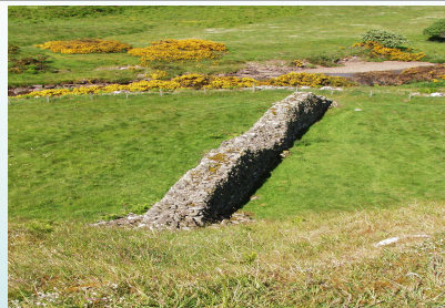
Wall A – Norse Foundation
