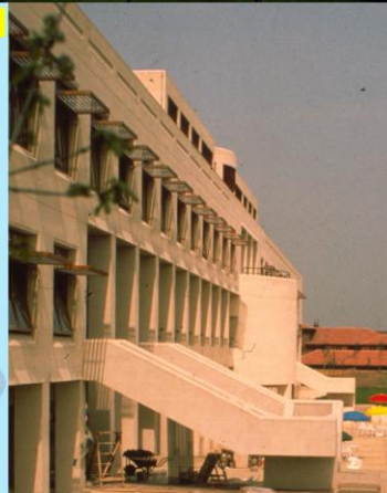
NFU Mutual and Avon Group HQ, mixed-mode head office, completed 1983, designed when at FRJM Refurbished by others, 2006, without adding air conditioning © Building Services Journal
