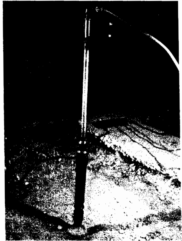
Figure 3.4 Single legged Pneumatic Tamper used on Subgrade
