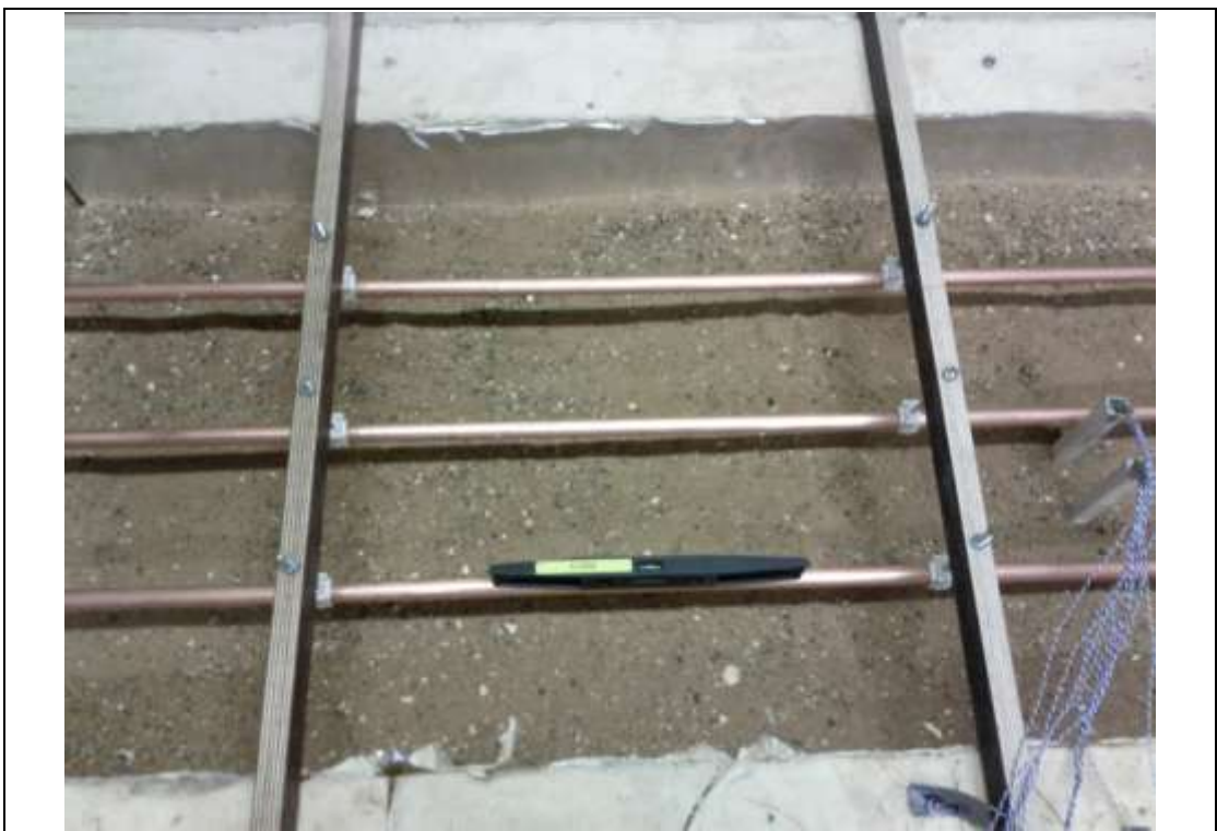
Figure 5-7 Supporting and levelling the collector pipes
