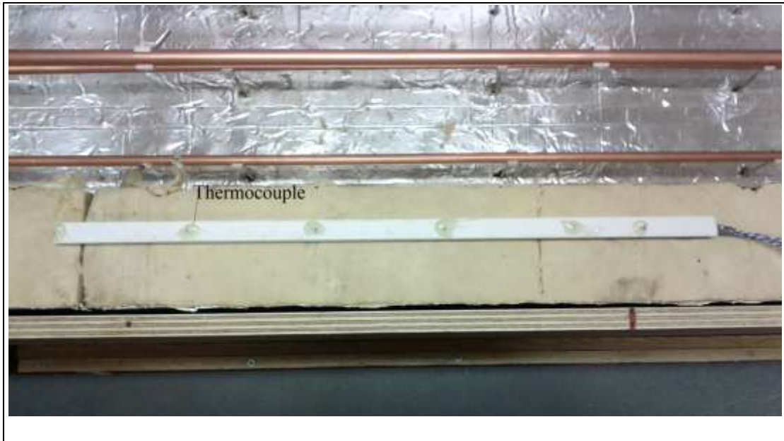
Figure 5-8 Thermocouples were fastened on a conduit
