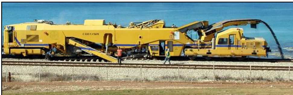
Figure 2.7 A ballast cleaner in action
