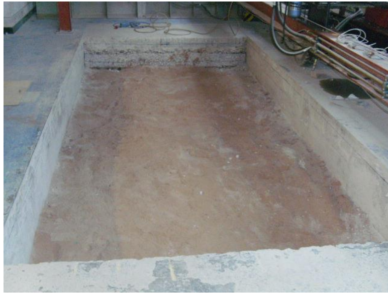
Figure 7.6: PTF Subgrade and capping
