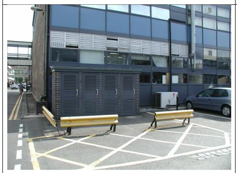
Gas storage at the side of a busy road - this storage facility has a lightweight roof, louvered doors and open grilled steel door to either end.
