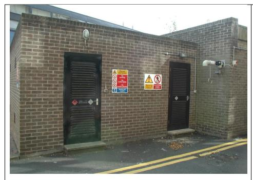
This photograph illustrates partial ventilation and potential pressure relief by the fitting of secure Louvre doors to the storage area.
