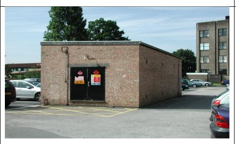
This store has a roof which is designed to relieve a build-up of pressure in an explosion.
