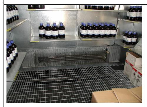
This shows the storage area for flammable materials in containers ready for issue - the floor is bunded, and the unit is well lit. Note the flame proof heater fitted to the wall.
