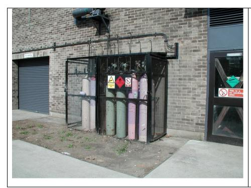
Another gas facility in a less used area - this is more open to the weather, but has a solid lightweight roof.
