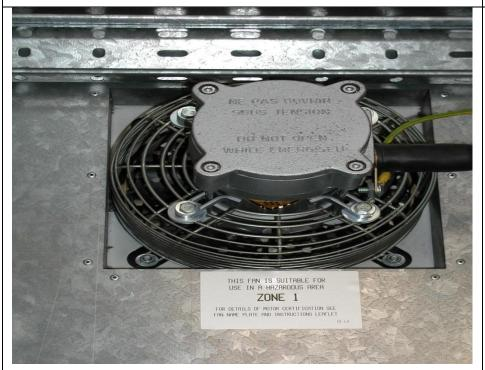
The high level fan fitted in the storage area - it is marked with a label on the wall of the store as being suitable for zone 1 use.
