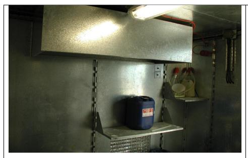
Decant and dispense area of the bulk storage area - built to the same standard as that shown above, but used primarily for accumulation and bulking of waste solvents, including flammables - the hood is exhausted via an externally mounted fan stack, controlled from outside the unit.
