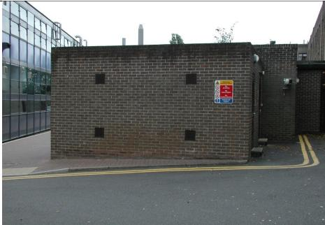
Side view of the store above showing adequate unobstructed crossventilation grilles.
