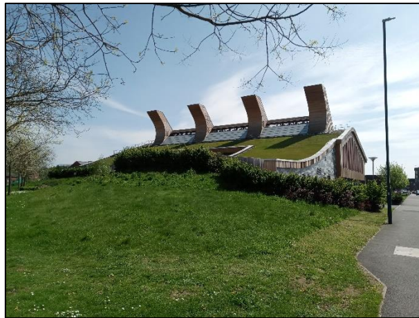
Figure 8 – Roof of GSK Carbon Neutral Laboratories for Sustainable Chemistry building
